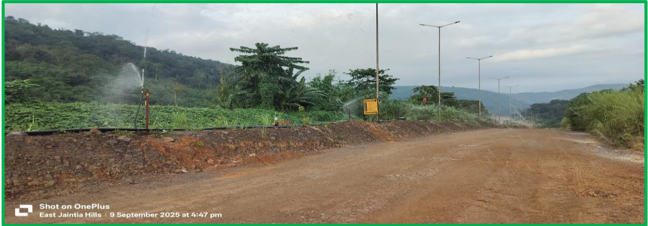
Water sprinkling through auto sprinklers
