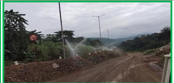
Water sprinkling through auto sprinklers
